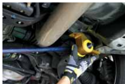
TO INSTALL THE ALK, YOU NEED TO DROP THE STOCK FRONT SUBFRAME SUPPORT, PRY THE FRONT CONTROL ARM DOWN, CHANGE THE BUSHING FOR THE ALK, AND THEN USE THE SUPPLIED SPACERS TO KEEP THE SUBFRAME SUPPORT FROM CONTACTING ANYTHING. A LIFT REALLY HELPS HERE.
