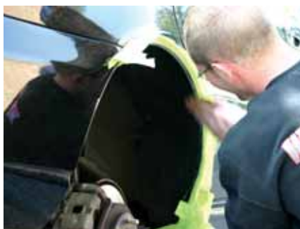
TO INSTALL THE ALK, YOU NEED TO DROP THE STOCK FRONT SUBFRAME SUPPORT, PRY THE FRONT CONTROL ARM DOWN, CHANGE THE BUSHING FOR THE ALK, AND THEN USE THE SUPPLIED SPACERS TO KEEP THE SUBFRAME SUPPORT FROM CONTACTING ANYTHING. A LIFT REALLY HELPS HERE.
